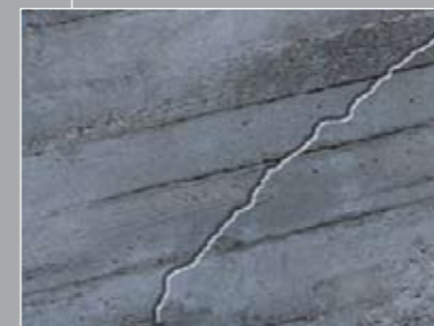
Structural Crack and Void Repair
