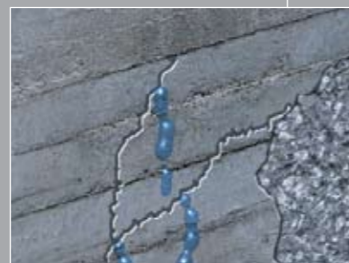
Surface Sealing of leaking Concrete Structures
